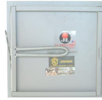
SPRING-ASSISTED CLOSING OF FD PANELS
